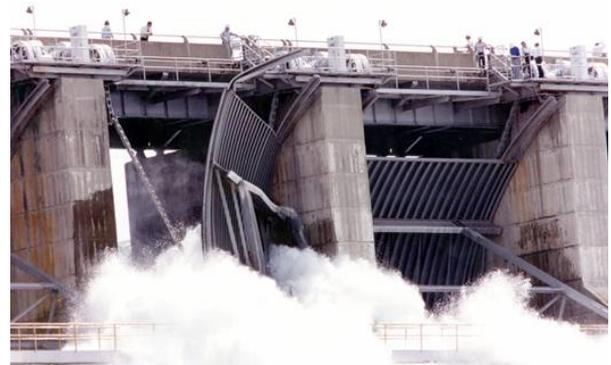
Figure 1: Tainter gate failure of an 87-ton gate at the Folsom Dam in California (USA) on July 17, 1995.
